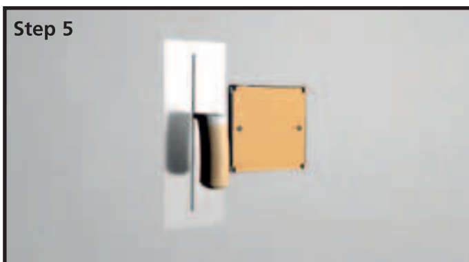
Step 5 Plaster, paint or tile and prevent excess moisture and plaster entering the electrical fixing.
