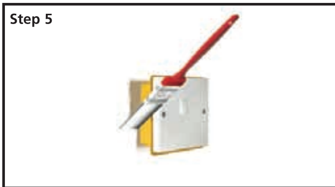
Step 5 Paint and prevent excess coming into contact with the electrical fitting to ensure a perfect finish.
