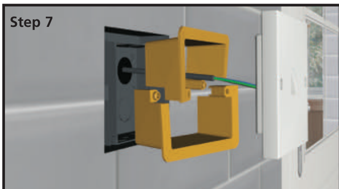
Step 7 Remove the fixing screws, unclip and remove the Safety Shield and reuse on your next electrical installation.
