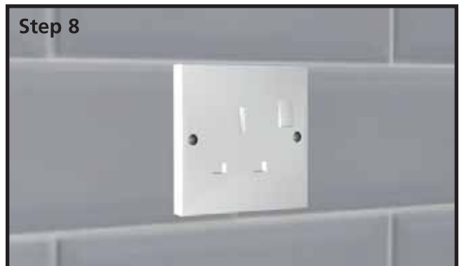
Re-install the fixing screws and complete final electrical safety tests and checks.
