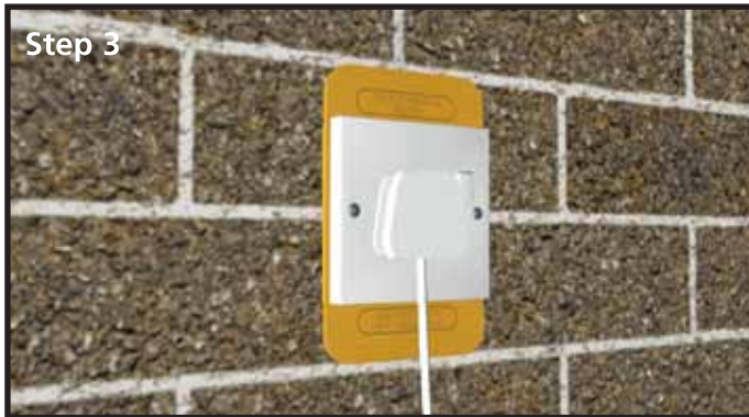
The electrical supply is safely maintained during the remaining building work and the electrician can leave site.
