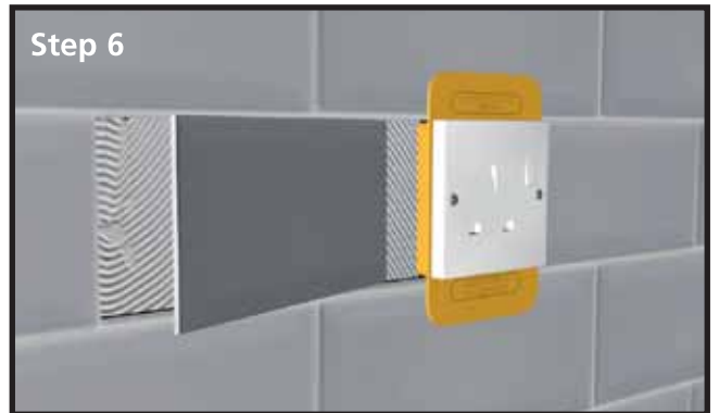
Tile with a clean edge to work from. The Safety Shield also ensures sufficient space is left to recess the fitting.
