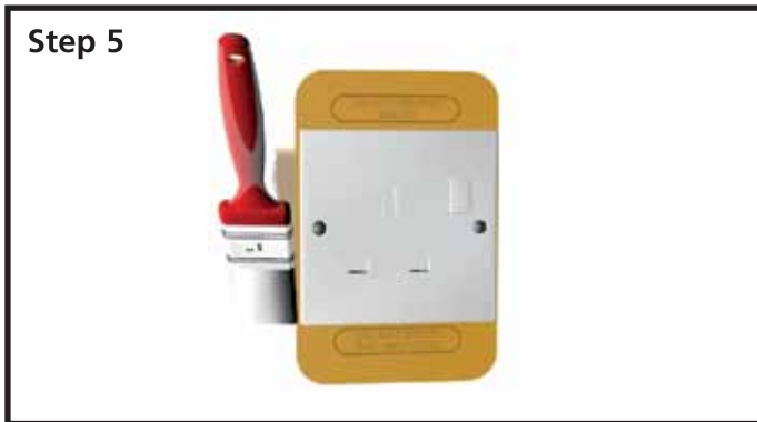
Paint and prevent excess coming into contact with the electrical fitting to ensure a perfect finish.
