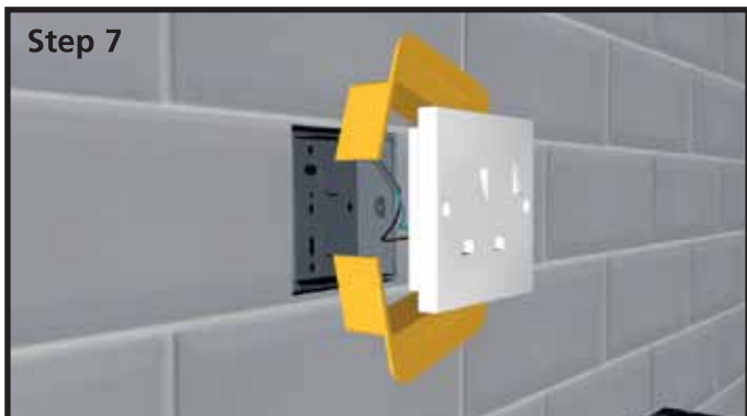
Remove the fixing screws and snap and dispose of the Safety Shield.
