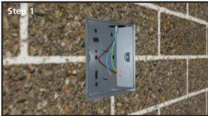
First fix - backbox and wiring installed as usual.
