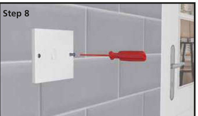
Step 8 Re-install the fixing screws and complete final electrical safety tests and checks.
