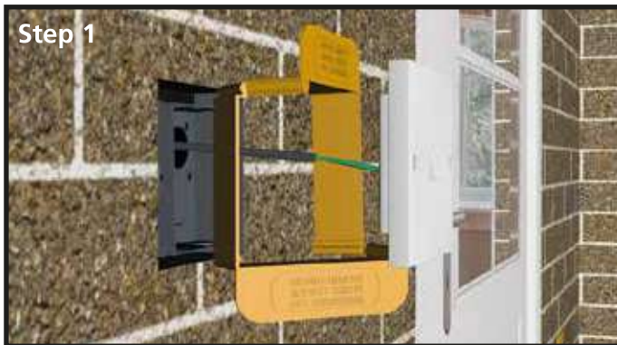
Step 1 First fix - unscrew the electrical fitting and clip the Safety Shield together so that the locating pins slide into the lugs.
